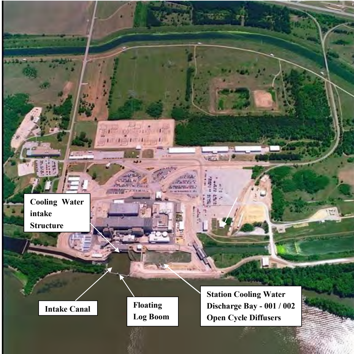
Figure D-3. Aerial View of Quad Cities Nuclear Station located on Pool 14 of the Mississippi Rive at River Mile 506.5 (LMS, 2005)
